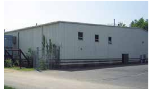
FSA production facility.
