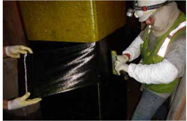
Syntho-Glass® XT was engineered to provide structural strength and leak sealing to prevent a refinery from an unexpected shutdown.
