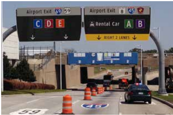
One of several arched trusses manufactured by Brookfield Fabricating found at the George Bush Intercontinental Airport in Houston, Texas.
