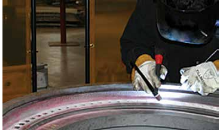
APG employee repairing industrial gas turbine engine.
